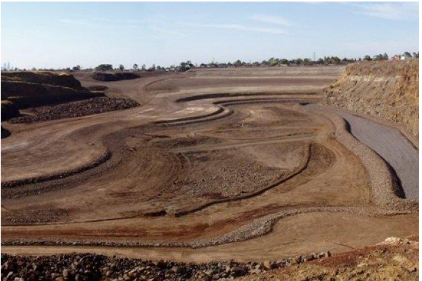
Northern View of Lake Contours after earthworks.
